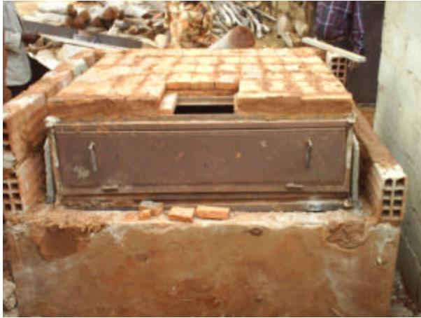
... exit out through the chimney that is located in the top course of the brick work.
