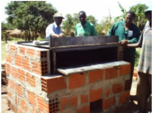
Three different ovens have been built in Mozambique since Nov 2003. The second and third version have been well received but the first version, which featured a baking compartment made of 2mm mild steel sheet metal, was not successful (see photo left). This was due to the different requirements of baking Portuguese rolls as opposed to 'loaf' type breads.
