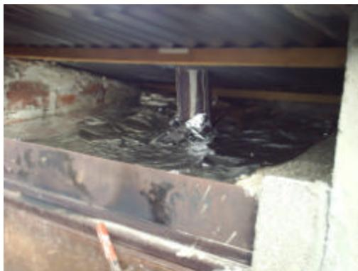
A layer of aluminum foil is placed on top of the vermiculite. More vermiculite is used to hold the aluminum foil in place
