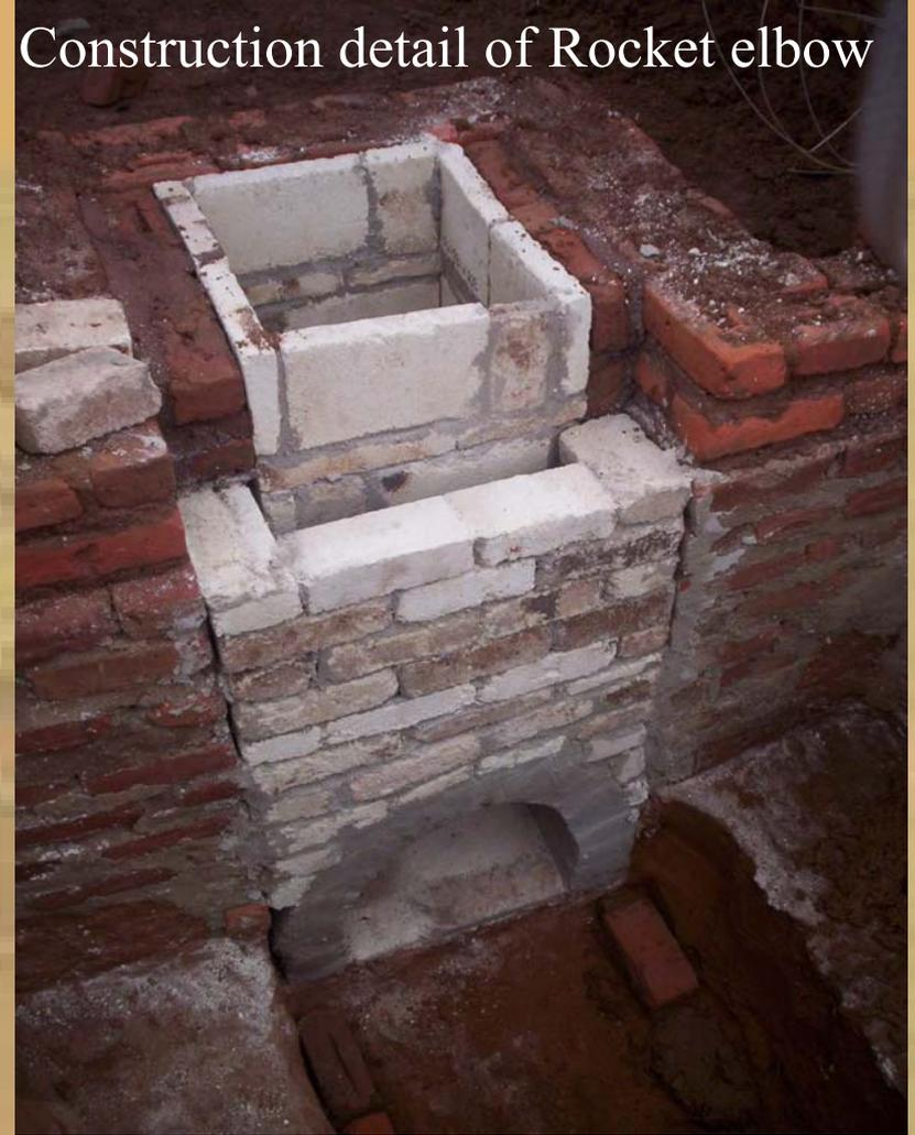
Combustion chamber made with high-
