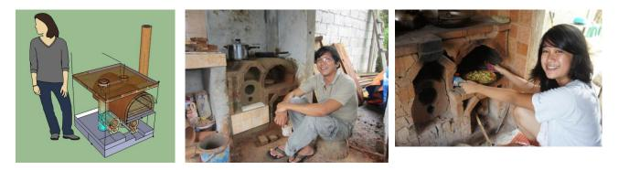
My 4n2 stove oven as planned, built and used. I used mostly bricks that I made and partly I bought at the hardware store. One of the stoves can serve the three cooking ports and the second stove will serve the oven. It took almost three months of drying until we finally inaugurated this project on February 2013 with a very yummy pizza which my daughter Mirasol prepared and enjoyed.
