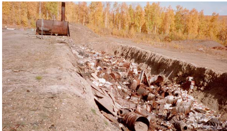
Figure A-2: Trench fill at Manley Hot Springs.
