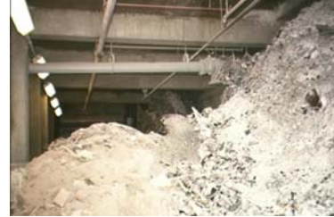
Figure C-10: Ash in storage vault.
