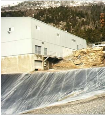
Figure C-2: Lined ash fill at facility.
