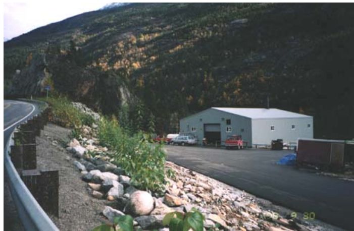
Figure C-1: Skagway materials handling and recycling facility with Thermal Oxidation System.
