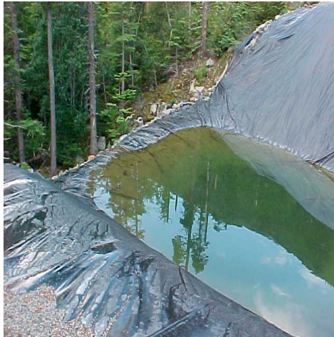
Figure C-13: Ashfill leachate at the ash fill.
