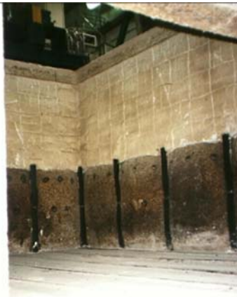
Figure C-6: Second floor view of the primary chamber.
