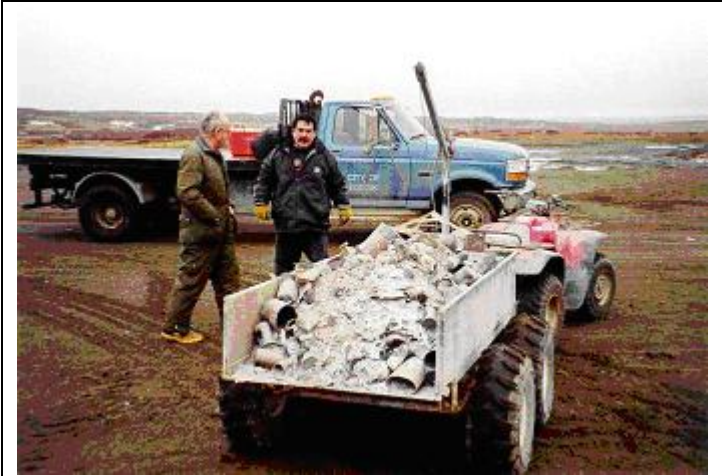
Figure B-5: Ash loaded for transport to ash fill.
