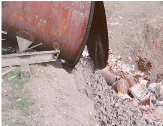
Figure A-9: Ash disposal into trench during clean-out.
