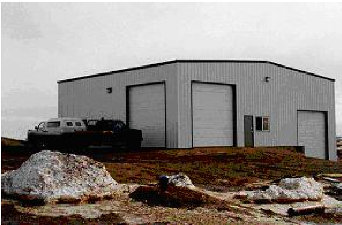
Figure B-8: Egegik incinerator building.
