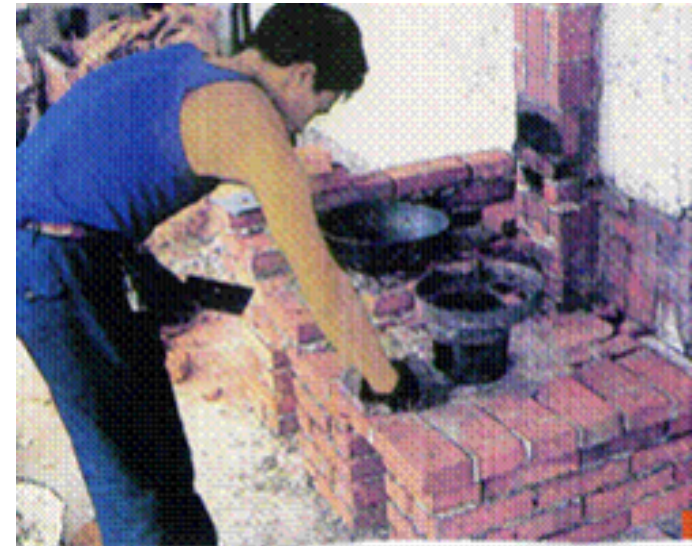
Farmer was installing the semi-commercial stove into the handwork stove.
