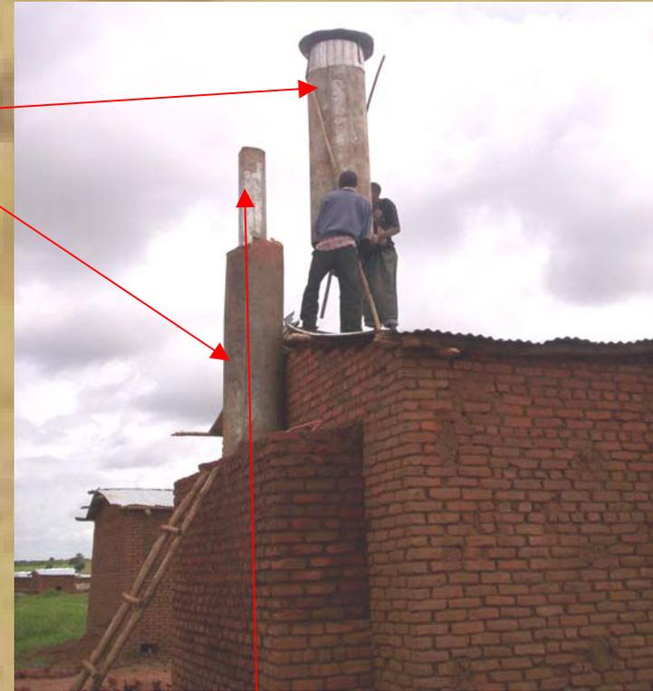
The external chimney is powered by the internal (30 cm) hot flue gas chimney. Ask Dr Larry for more info....
