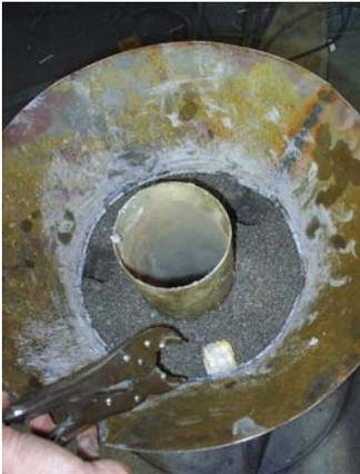
These will create a slot/opening for the pot legs to sit into. Let the mixture set overnight or for 8-12 hours, and then remove the blocks from the insulative mixture
