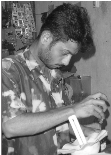
Figure 2 Installing solar lighting in a shop (photo: Kunal Mehta)
