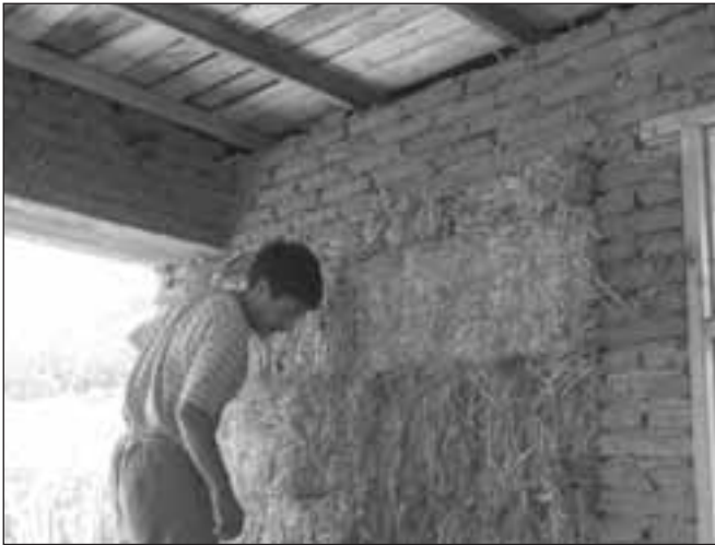
Figure 3 Straw-bale construction utilizes a waste product
