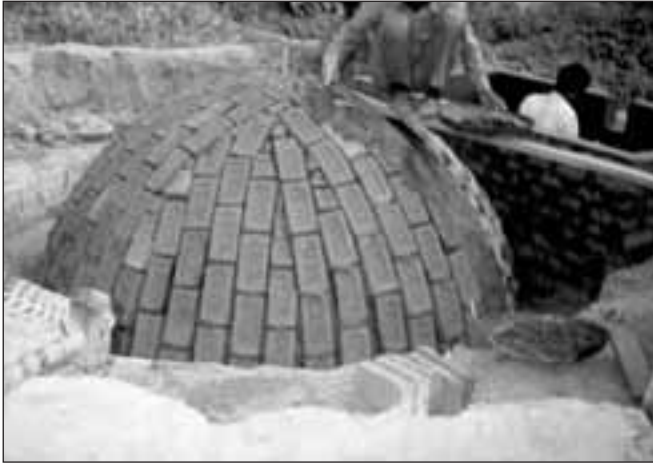
Figure 2 Biogas plant installation (photo: Rakesh Prasad)
