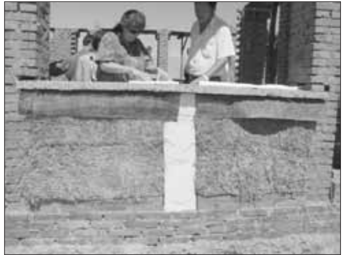
Figure 4 Building with brick and straw
