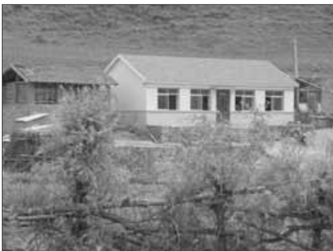
Figure 1 Typical straw-bale house
