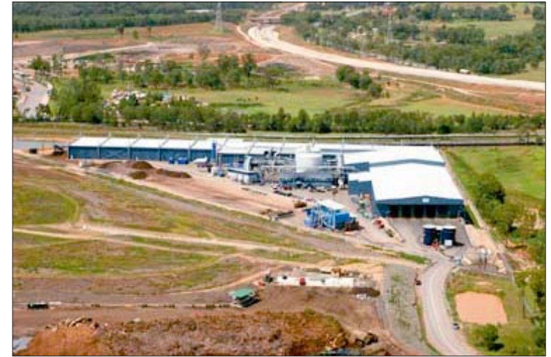
Global Renewables' waste management and recycling facilities at Eastern Creek, Sydney.
