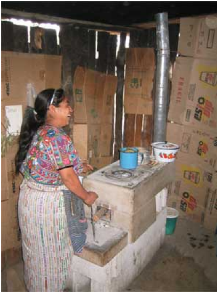
Improved Stove and Chimney Avoids Creosote Build Up in Rafters
