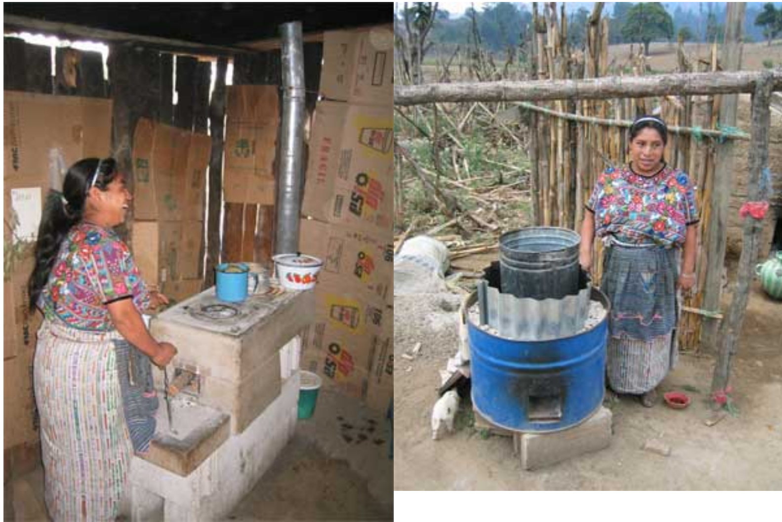
Improved Stove and Chimney Avoids Creosote Build Up in Rafters
