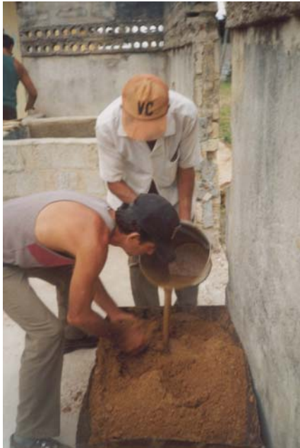
Finely ground biomass is mixed with clay....
