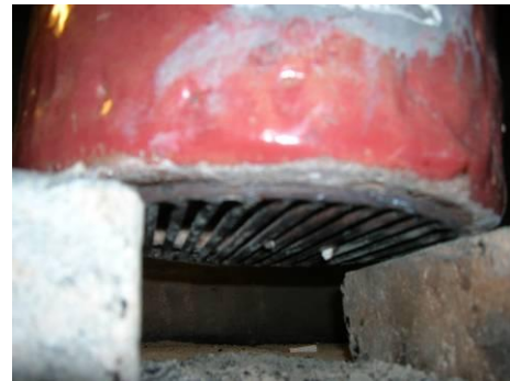
Grate under chimney to hold charcoal
