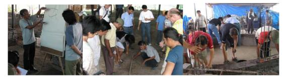
From day 6 up to day 9, the training took place in Mr. Bhuengwongyart's charcoal factory. Participants took part in the construction of different parts of lwate kiln – the floor, the wall, the chimney and the roof. Another hands on component of the training was on the process of wood vinegar production.
