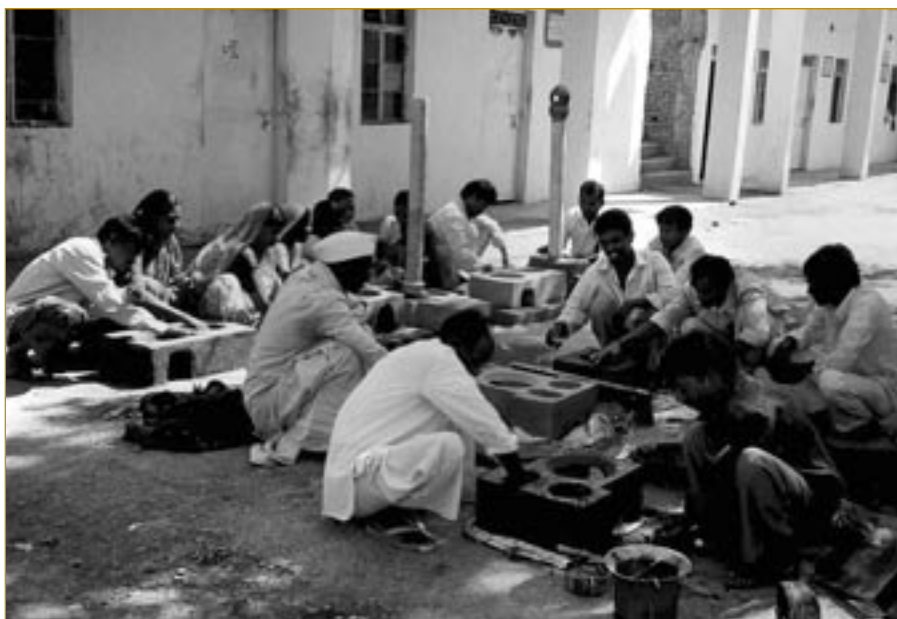
TRAINING ON MOULD-USE FOR STOVE CONSTRUCTION
