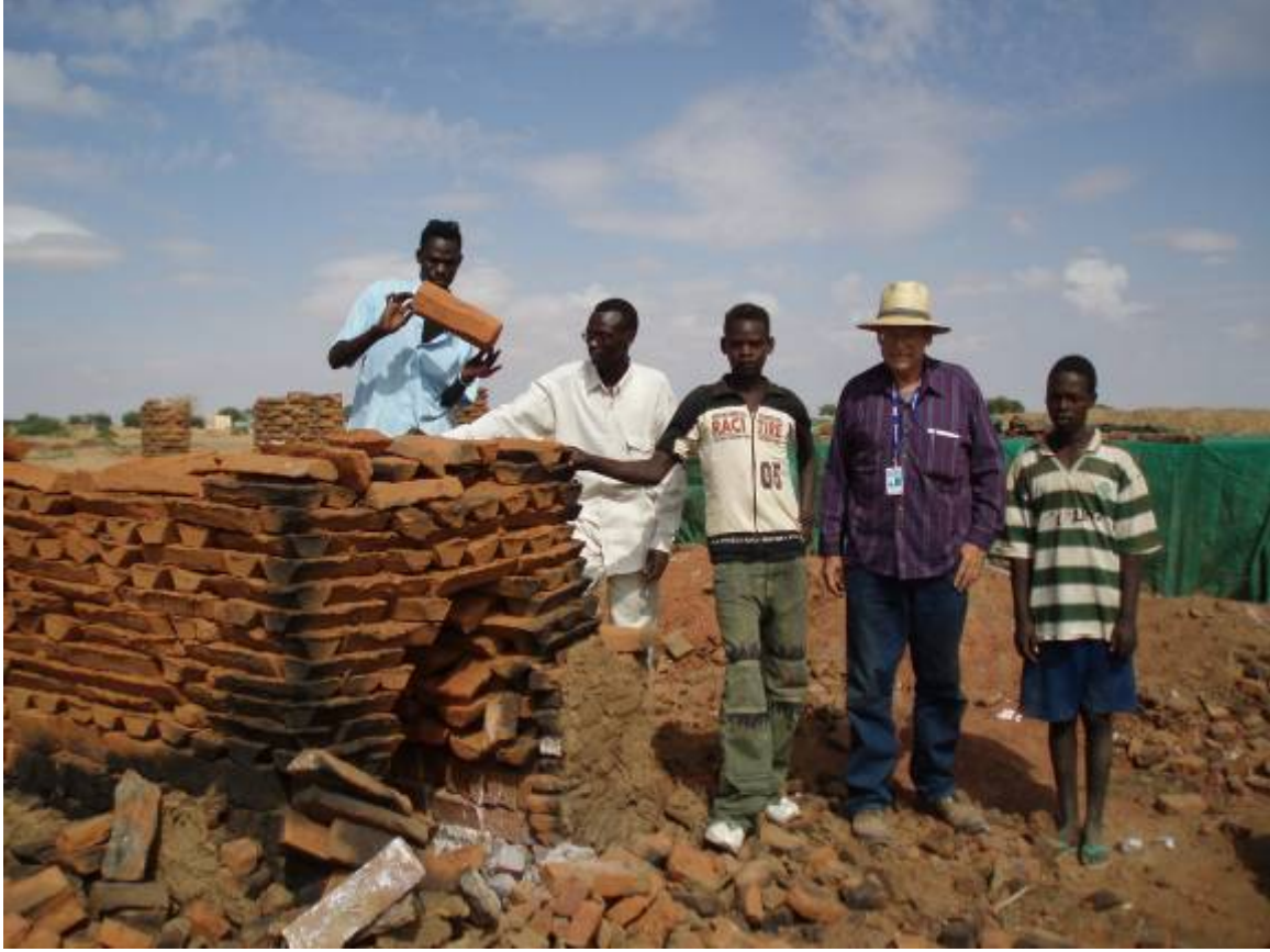
Our first batch of bricks has been successfully burned.
