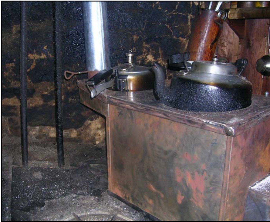
Stove with sunken water kettle and pressure cooker. The dimension of the two holes will accommodate most medium-sized pots, leaving only a minimal gap around the pot. On the left are the two vertical pipes of the back-boiler from the existing mud stove.
