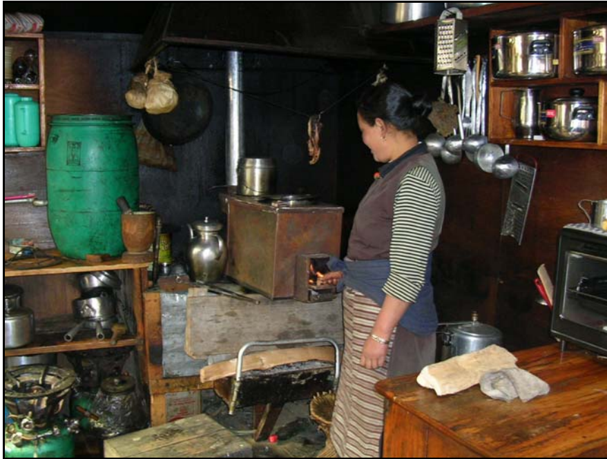
The new stove placed on top of the old mud stove and already in use.
